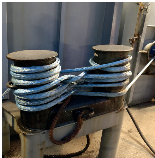
Puller uegnet for slep fordi Safe Working Load (SWL) mangler.
